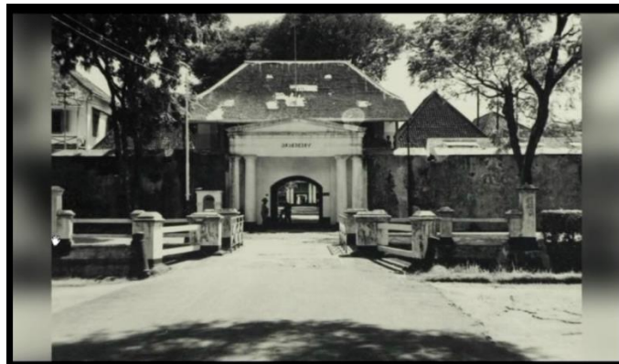
Gambar 4.1 Program “Garda (Bangunan Cagar Budaya)”
